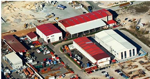
PK-PRODUCTION AND SERVICE FACTORY KUKULJANOVO
